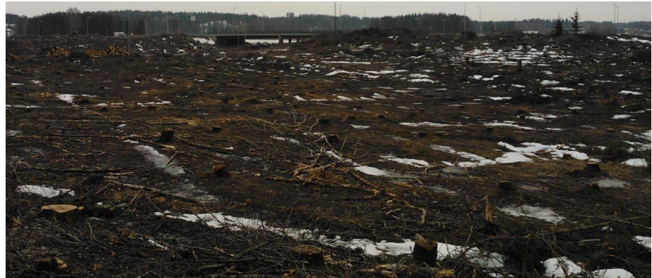
Situation before mass stabilization at project area
